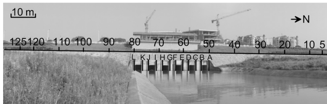
Figure 8. Illustration of the field test. Symbols A, B, C, D, E, F, J, K, and L in the figure indicate different sites on the load-bearing walls of steel bars. Right above the drainage culvert (profiles 50–80 m), site separation is 0.5 m, and on two sides of the drainage culvert (profiles 5–50 and 80–125 m), the site separation is 2 m.
